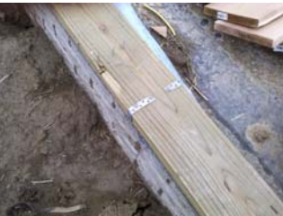
Anchored sill plate. At same site of house that slid off its foundation. Photo by NWS Des Moines, Iowa.
