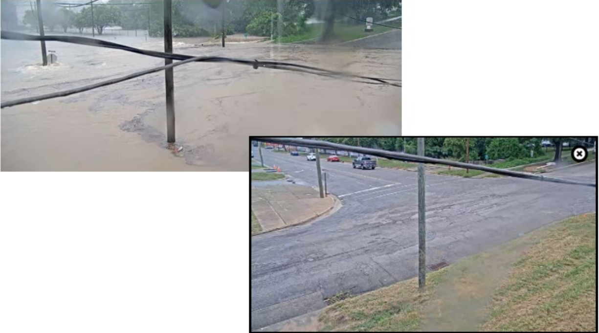
Figure 7. The intersection of Main Street and Whaley Street. The creek normally flows through a cement culvert underneath the intersection. In the picture, you can see the extensive flooding as the creek flows over the roadway and into the intersection. The flooding picture was taken during the record flood of 4 July 2022.
