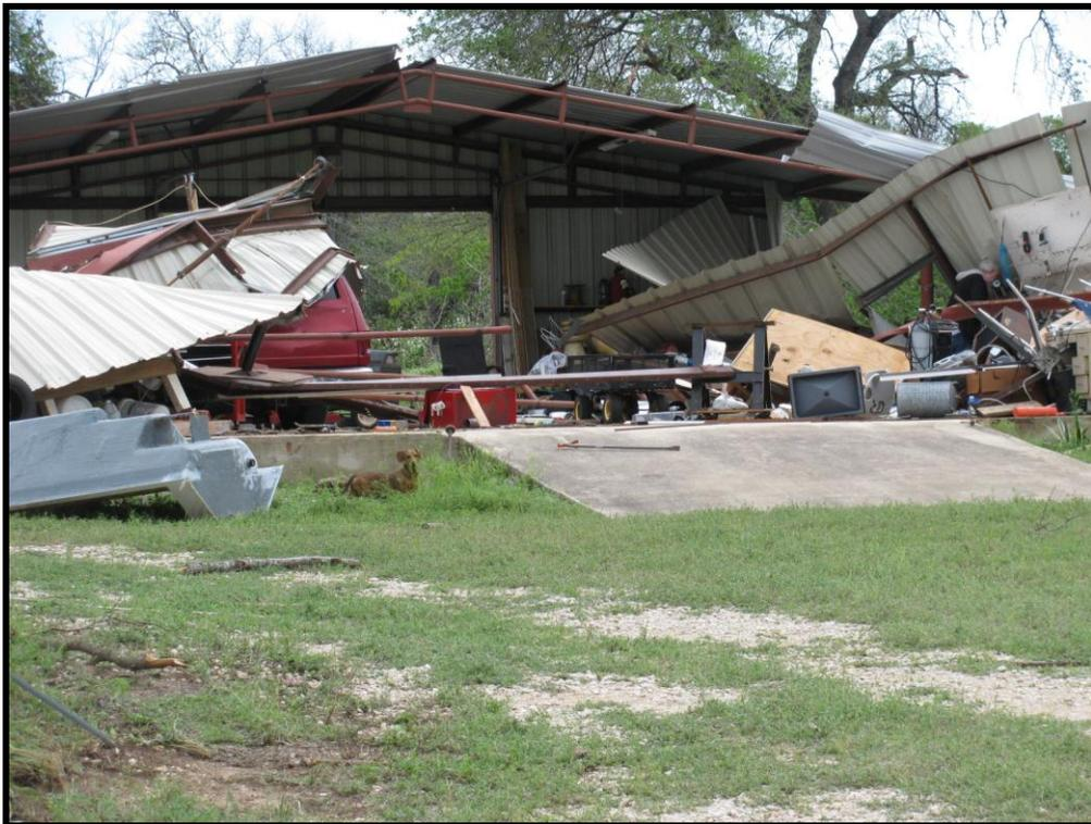
Figure 5. A steel frame shed severely damaged by the EF1 Tornado near Natalia, TX, on March 19, 2012.
