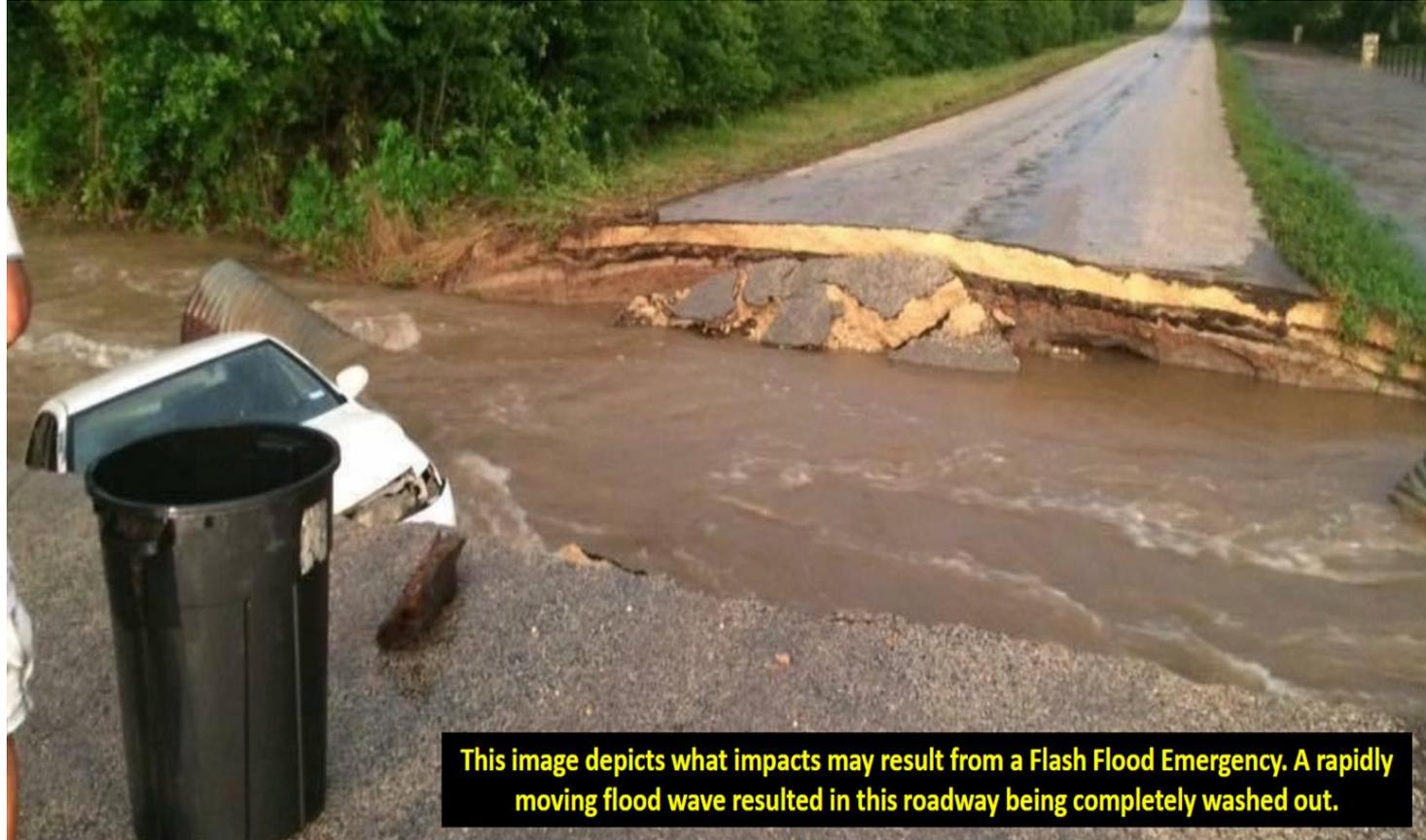
**This image depicts what impacts may result from a Flash Flood Emergency. A rapidly moving flood wave resulted in this roadway being completely washed out.**
