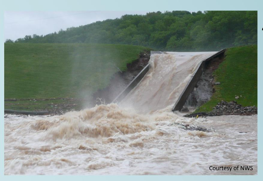
Significant flooding occurred due to high crests on major rivers. The table above lists the affected rivers in Kentucky. Dunham Lake Dam in Metcalfe County (above) experienced structural damage and almost breached due to high water levels. River flooding also affected county roads near river beds, shown below (Roseville Road, Barren County).
