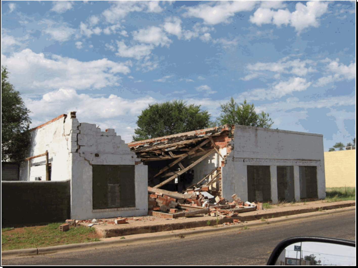
Several buildings suffered heavy damage as thunderstorm winds measured up to 93 mph impacted Morton (Cochran County) during the late evening of the 17th. Photo courtesy: Danny Wiseley - Texas Tech University West Texas Mesonet.
