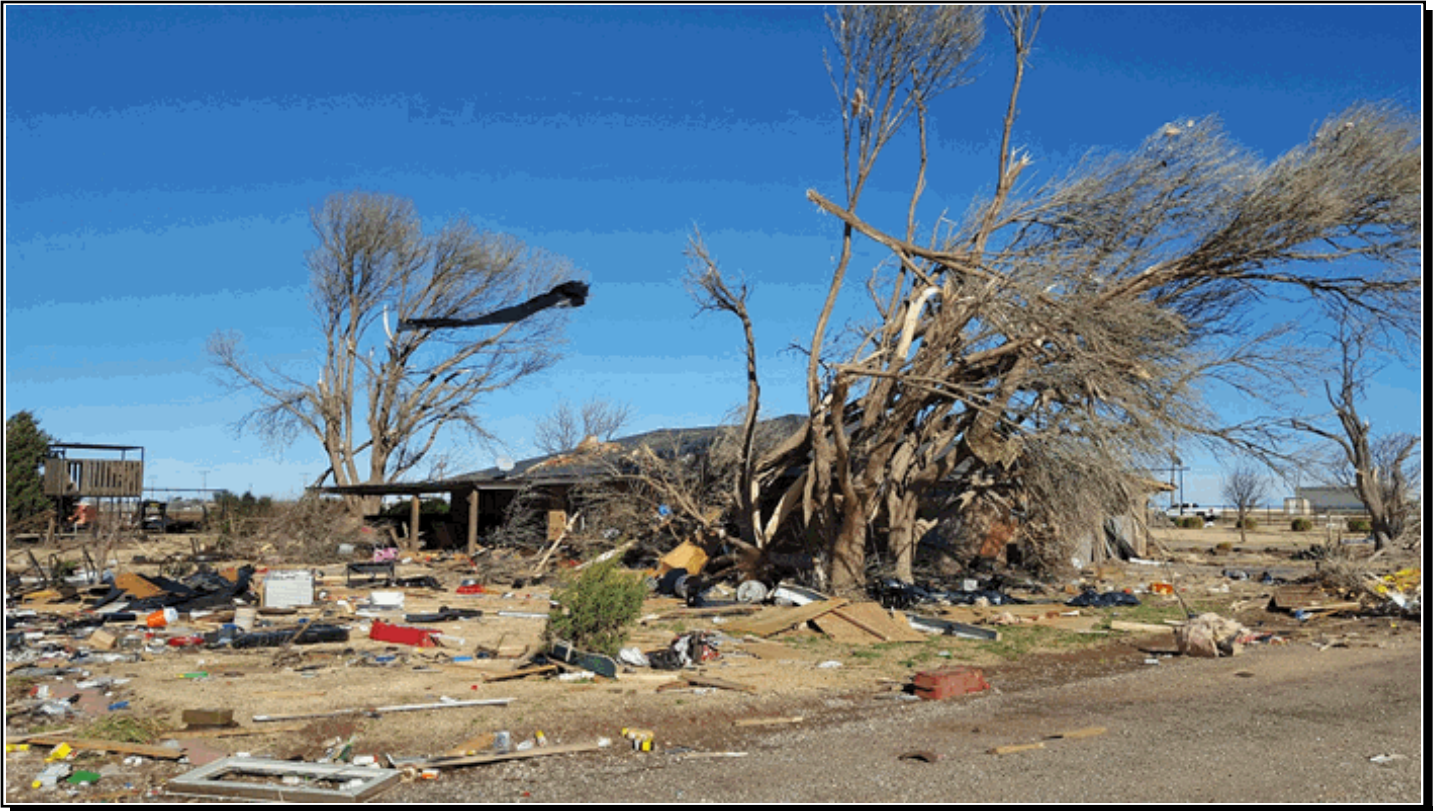
Damage to a house near Anton, TX caused by an EF1 tornado. Photo from the NWS Lubbock damage survey.
