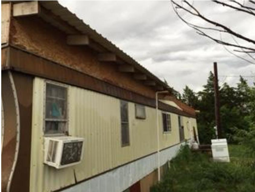
Figure 1: Wind damage to roof.
