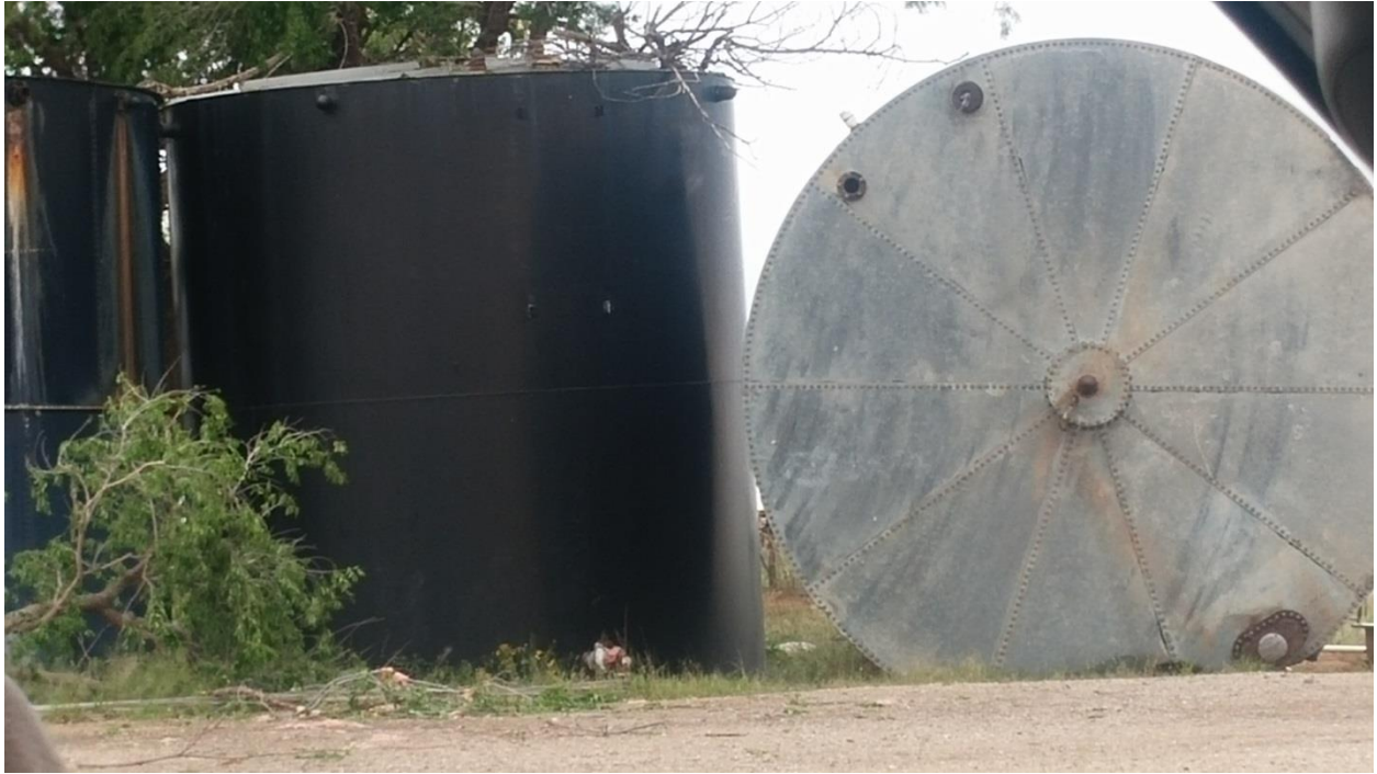
Figure 14 – Overturned large tank (Courtesy of David Hennig).
