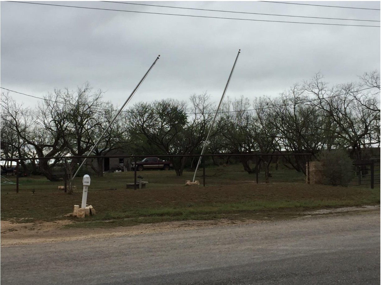
Figure 13 – Bent flagpoles (Courtesy of Mark Strobin).
