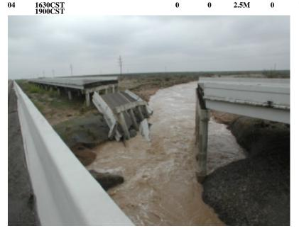
A bridge along Interstate 20 just east-northeast of Toyah over the normally dry Salt Draw failed Sunday evening. This failure was the result of fast-moving flood waters originating from previous heavy rainfall over the Davis Mountains. Hydrologists also credited a residual flow of water through the draw from the Toyah dike break early Sunday for contributing to the gradual process that caused
