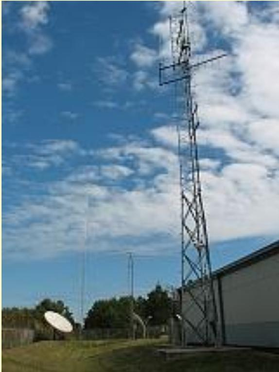
**GAP Voyager, CL33 rotatable beam & VHF tower**
