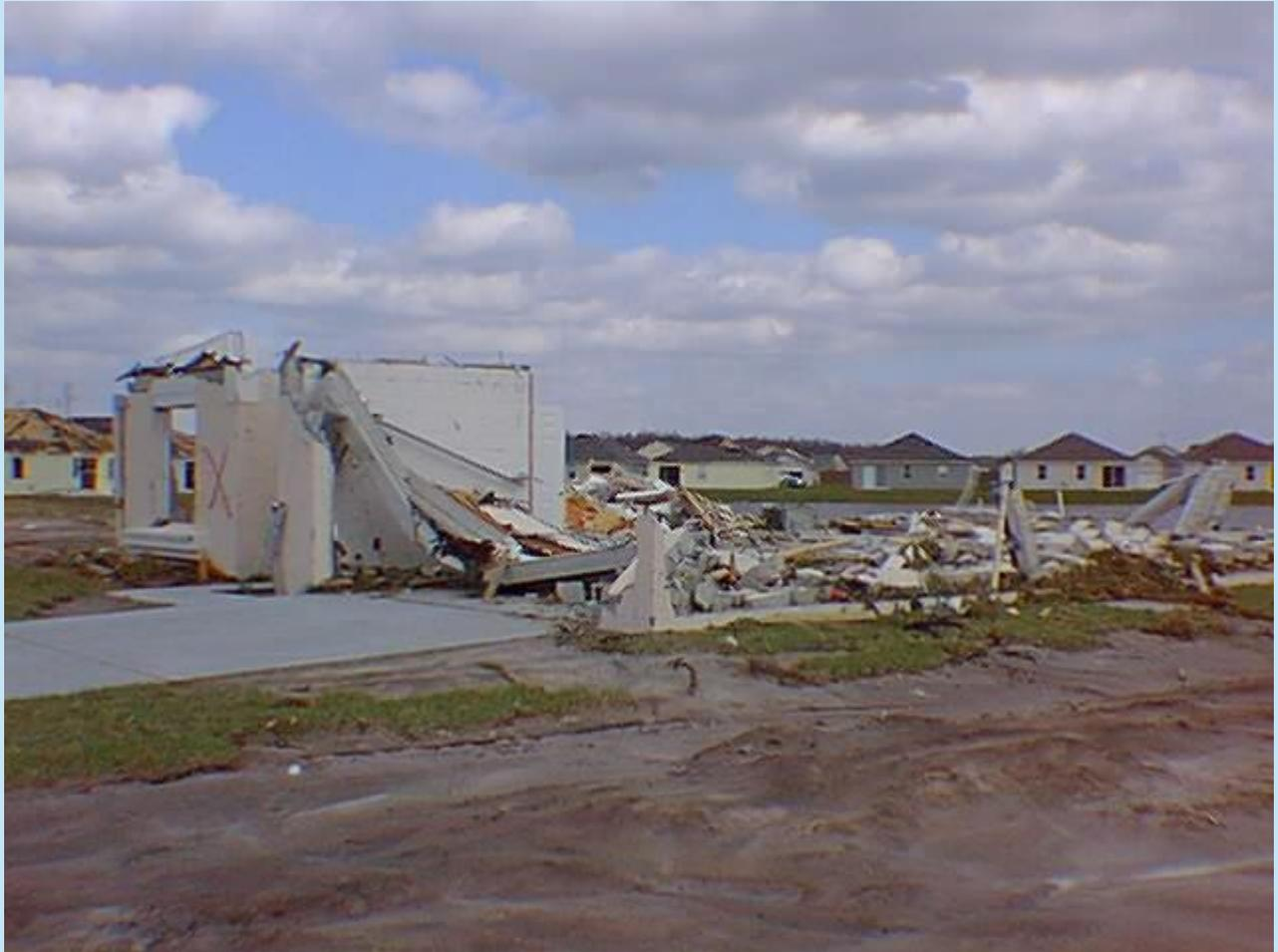
**All that is left of what was a brand-new concrete-block and stucco home, Structure left standing is front-door entryway and one partial wall with a window. This subdivision was directly across the Florida Turnpike from the RV Park, where damage photos above were taken.**
