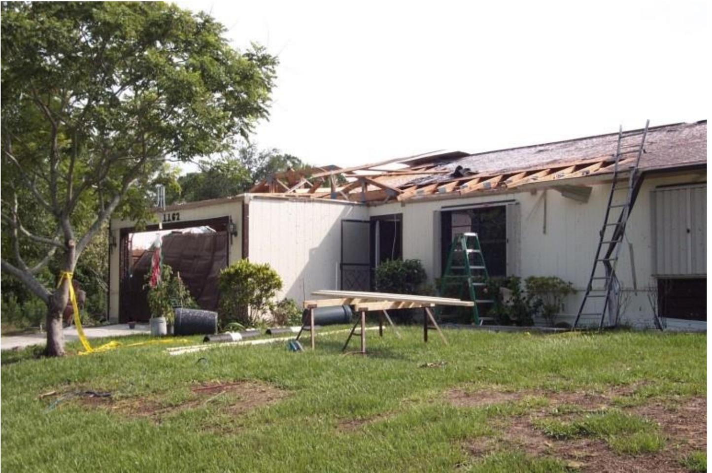
**Significant roof damage (F1) to home.**
