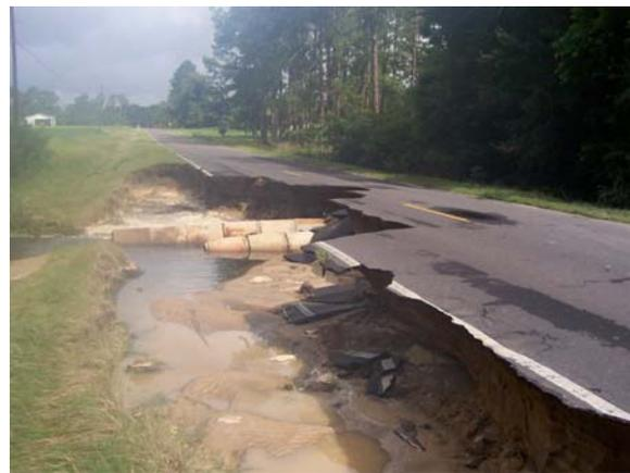
Figure 8. Photograph of Flash Flood induced culvert damage in Moultrie, GA. Photo courtesy of Russell Moody, EMA Director, Colquitt County, GA.
