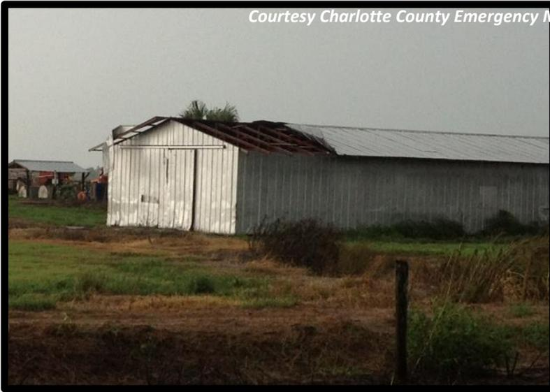
This photograph shows damage to a roof of a metal outbuilding at a sod farm on 31 caused by straight line winds.
